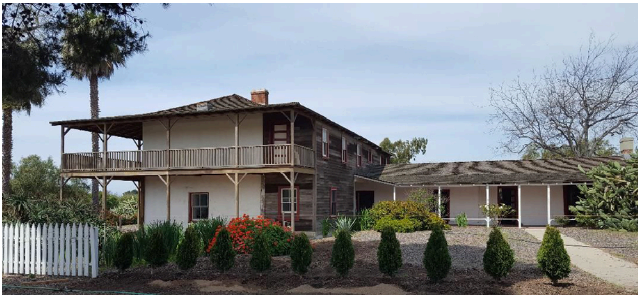
Figure 3. Las Flores Adobe, a former mission asistencia and later rancho structure that demonstrates how colonial settlement expanded along natural coastal and valley corridors.
