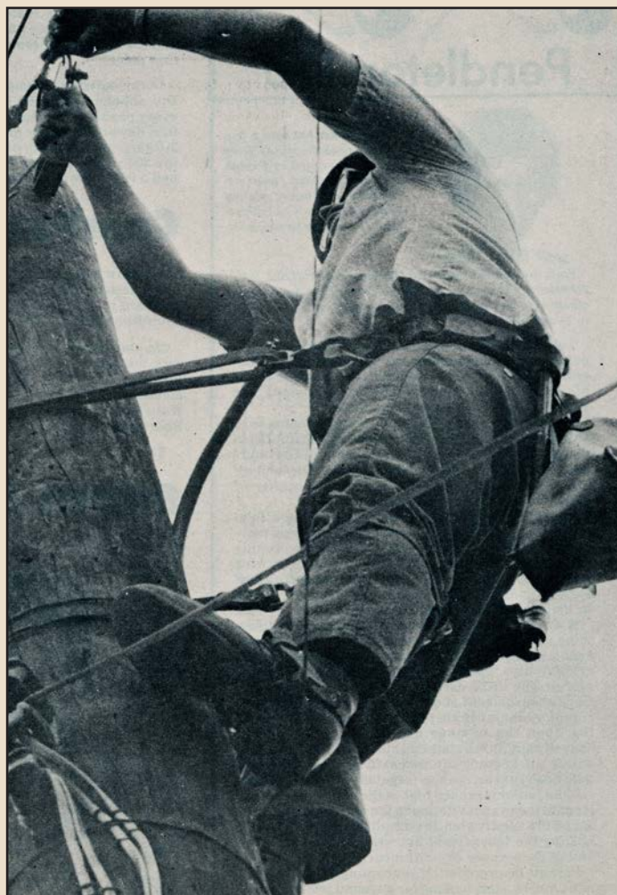
Miles of electrical lines came down as the order to shut down was passed.
