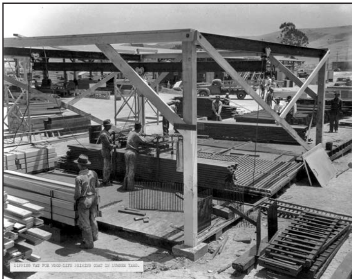
Dipping vat for wood-life priming coat in lumber yard
