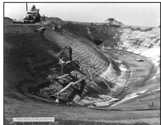
Gunite machine at work on reservoir
