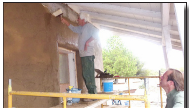
Exterior restoration of Las Flores Carriage House
