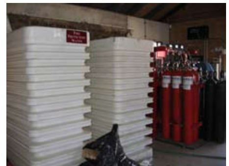
The white containers that are filled with water and the red nitrogen canisters.
